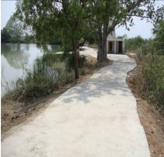
CC Road at Negi Para in Nariyara village
